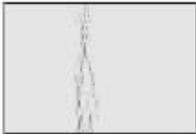
图 3 单轴受拉试件最终裂缝 Fig.3 Final cracks of specimen subjected to uniaxial tension
