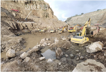
(a) 左岸高陡坡处边坡挡墙
