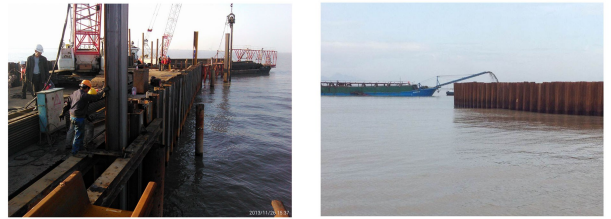
(a) 钢板桩打设
